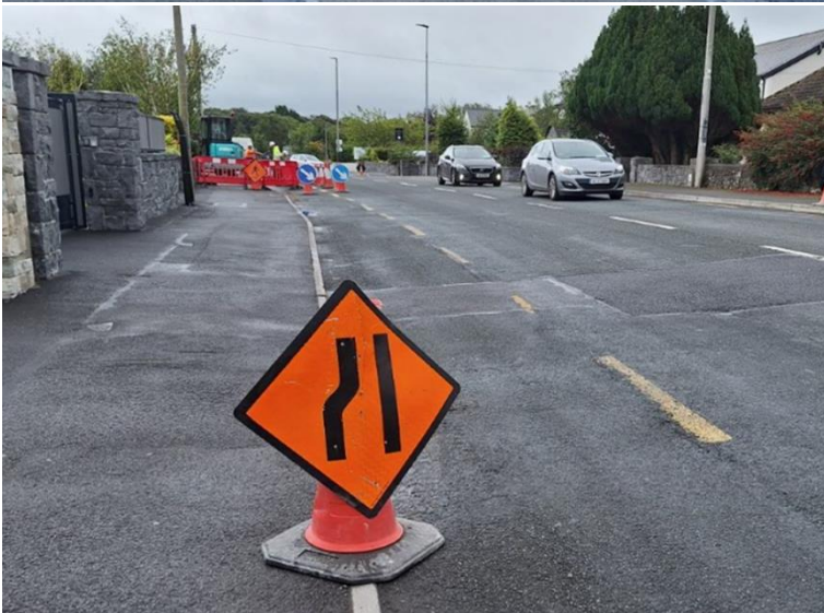
SLIT TRENCHES FOR LIDL PEDESTRIAN CROSSING ORANMORE
