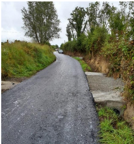
(RI) RESTORATION IMPROVEMENT, AT GARRAFINE - DBM WORKS IN PROGRESS
