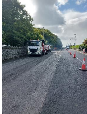
N67 During works
