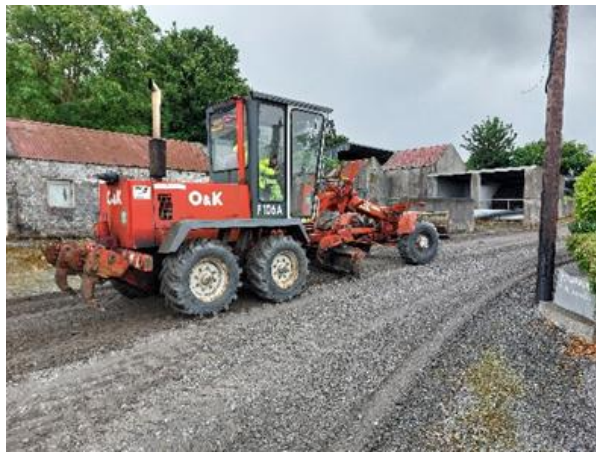
ROAD RECYCLING CLADDAGH WEST
