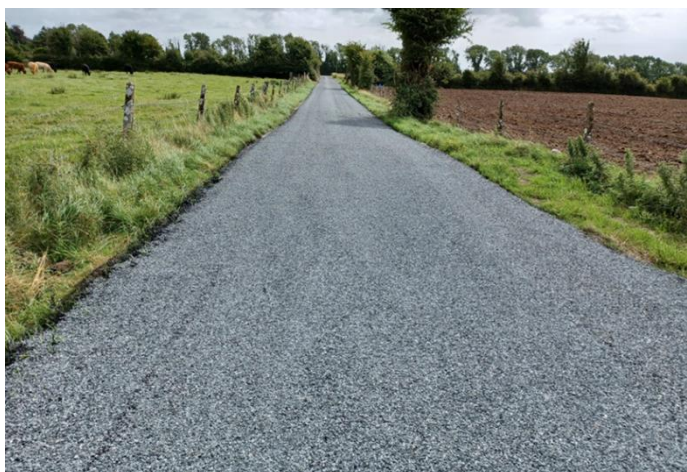
ROAD RESURFACING WORKS COMPLETED AT MULLAGH BEGUNDER A LOCAL IMPROVEMENT SCHEME
