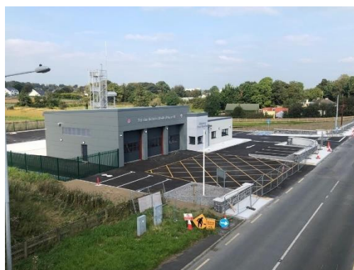
NEW FIRE STATION ATHENRY
