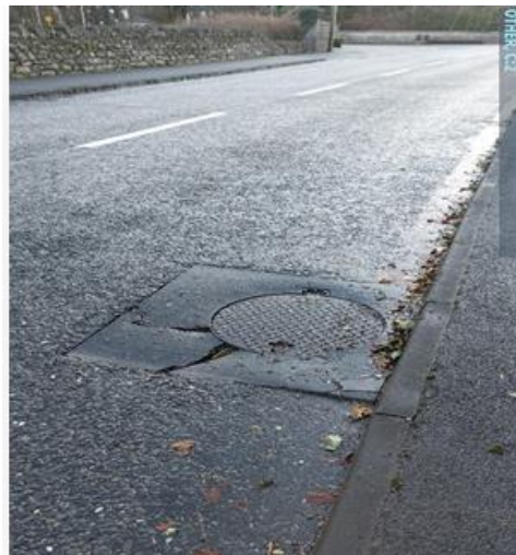
N67 BEFORE WORKS
