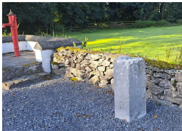
MILESTONE MARKER UPGRADE WORKS – COOLE PARK
