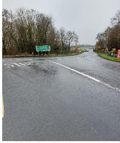
N63 BEFORE WORKS
