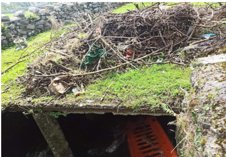
ATHENRY PLAYGROUND BRIDGE CLEARING
