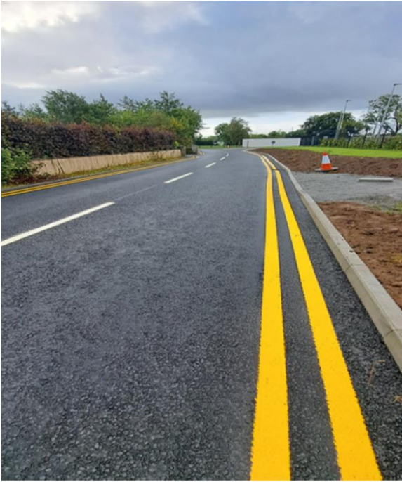
CRAUGHWELL NATIONAL SCHOOL – NEW KERBING, DRAINAGE & OVERLAY WORKS
